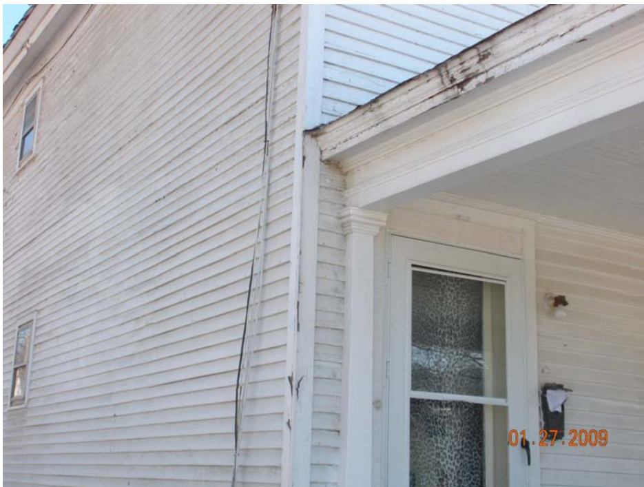
“A” side: 2 nd floor eaves over porch
