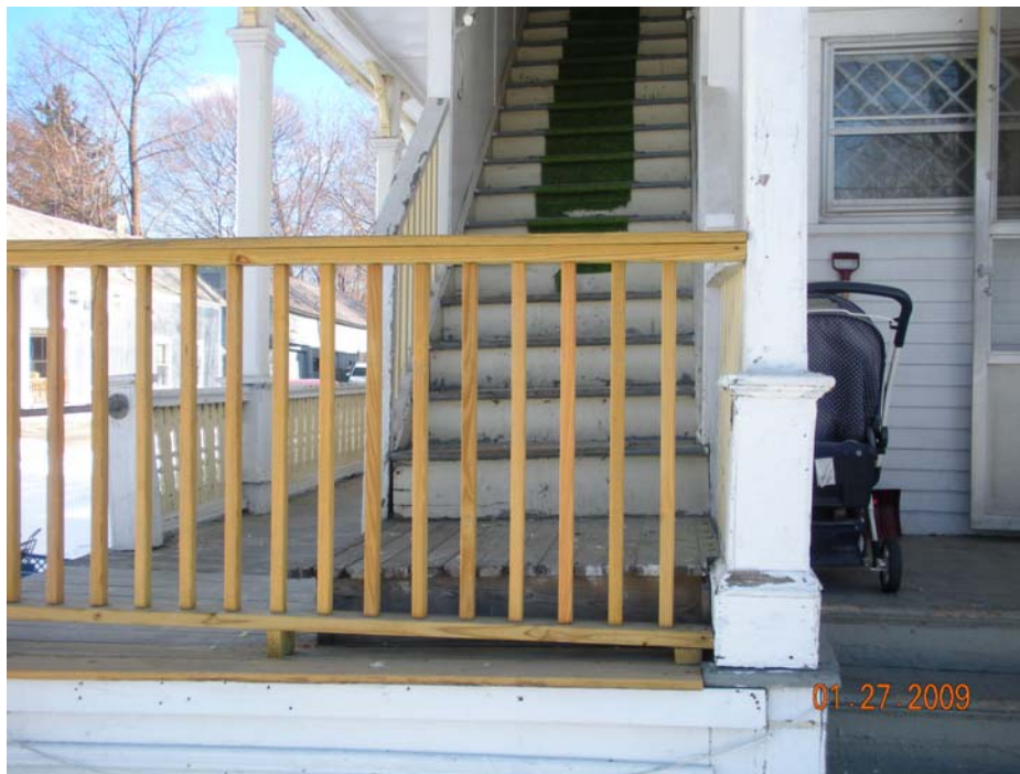
“A” side: front porch and stairs to 2 nd floor
