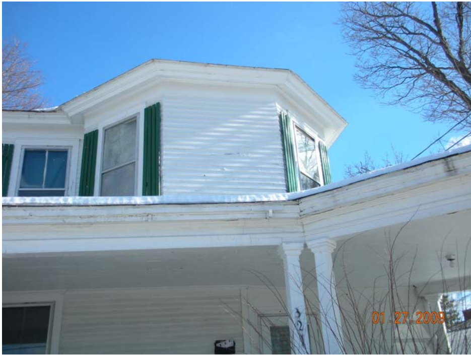
“A” side: porch and eaves; “A” side 2 nd floor wall
