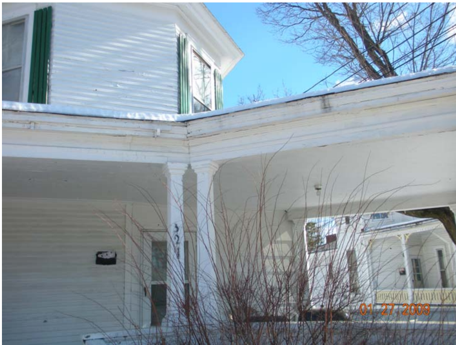
“A” side: porch at 321 School Street
