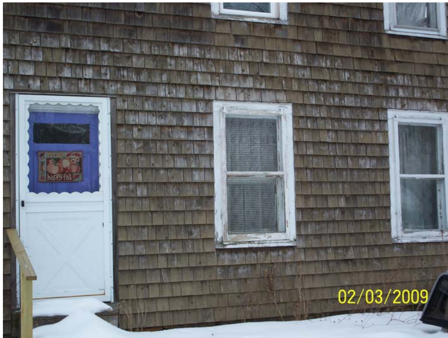
“A” side: building exterior
