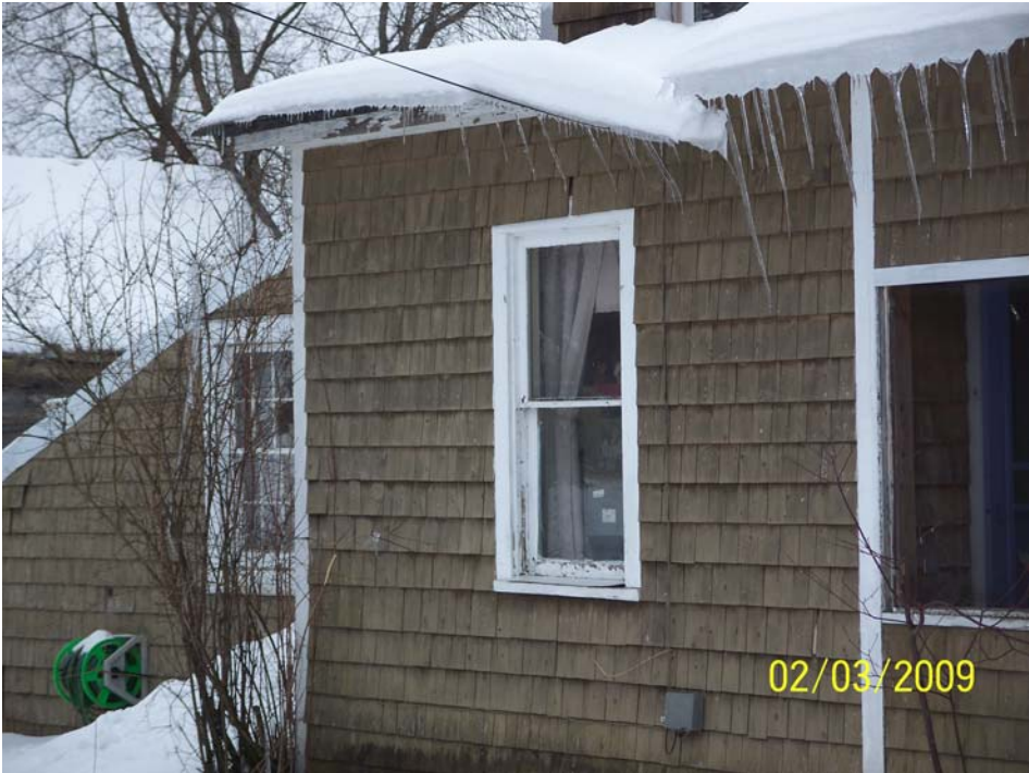
“D” side: building exterior
